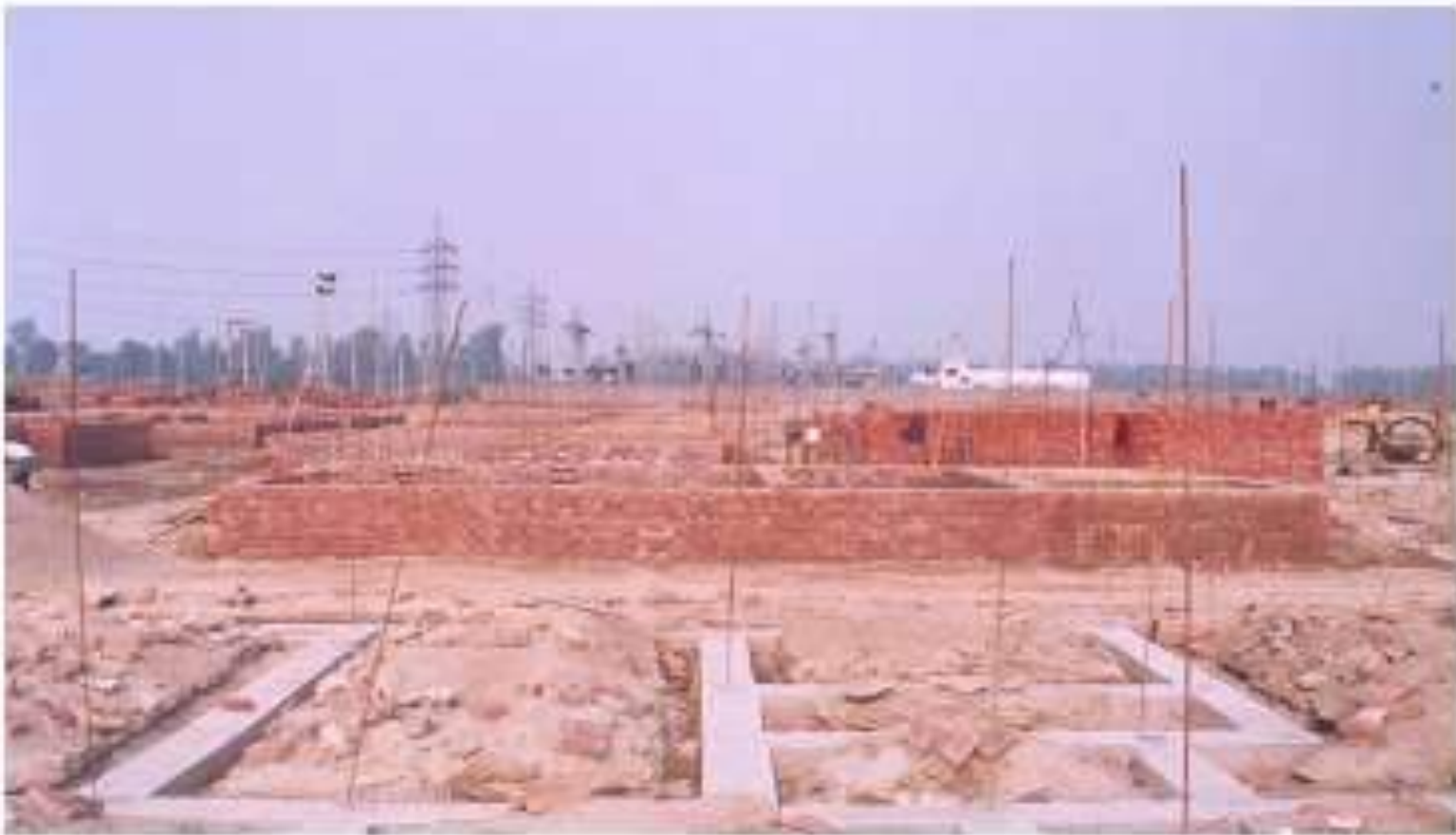
Grade Beam & Vertical Reinforcement (for Earthquake Resistance)
