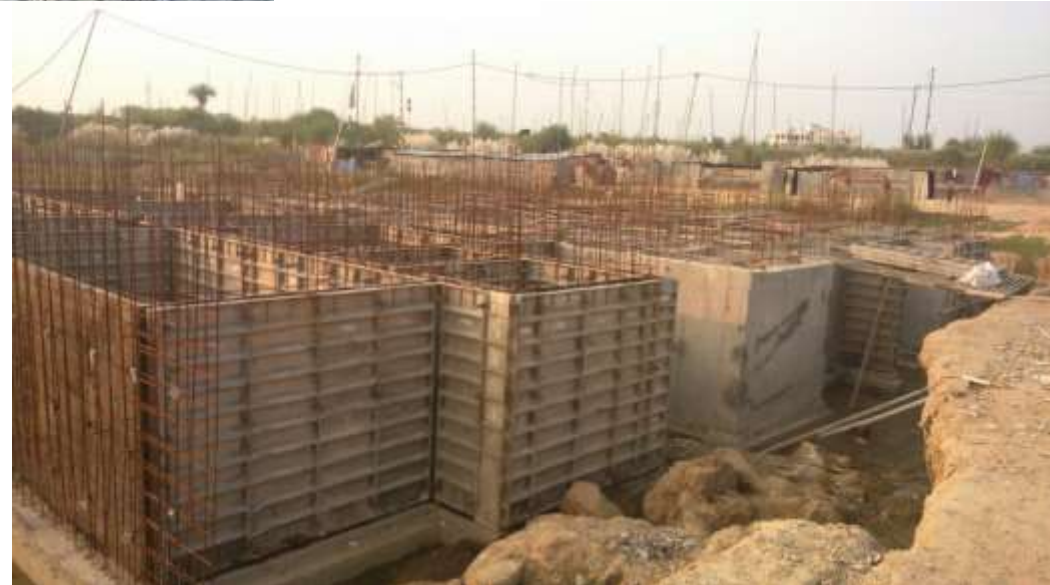
Form work for Walls below plinth
