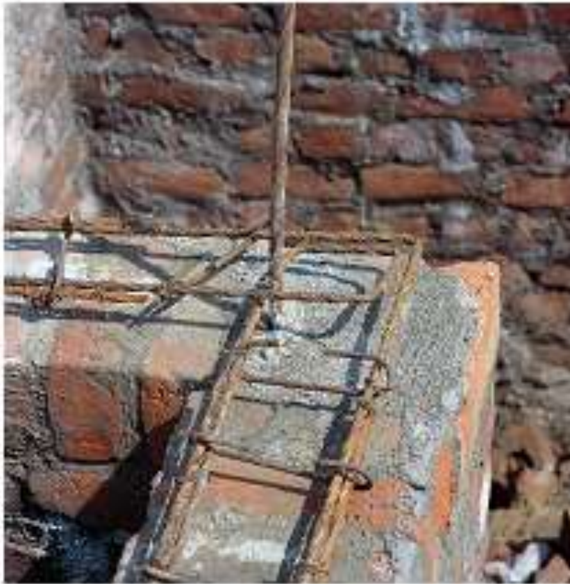
Vertical Reinforcement L - Junction
