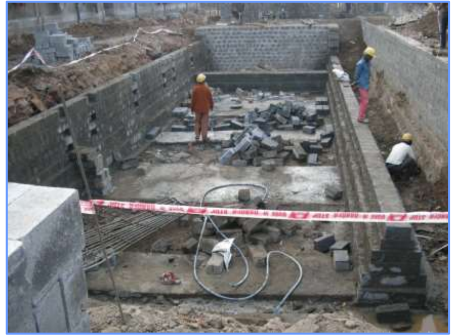
Foundation at Vapi site with Concrete Blocks
