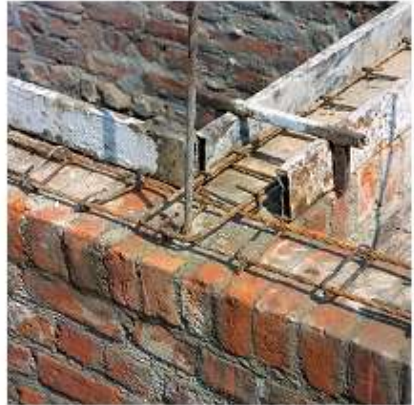
Vertical Reinforcement T - Junction
