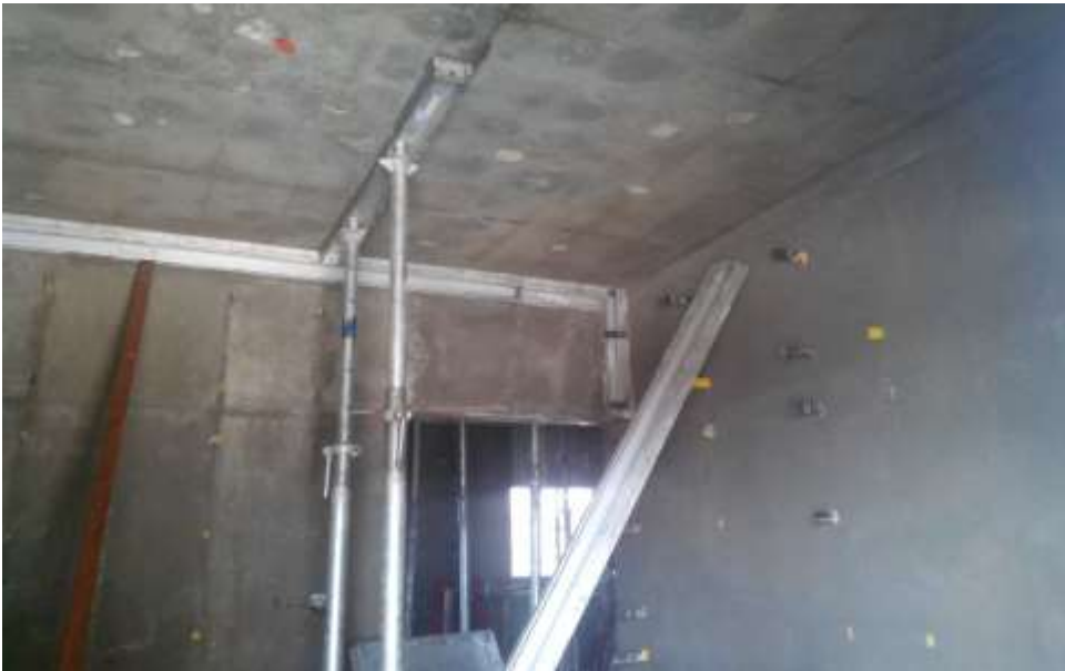
Ceiling view after removal of Formwork
