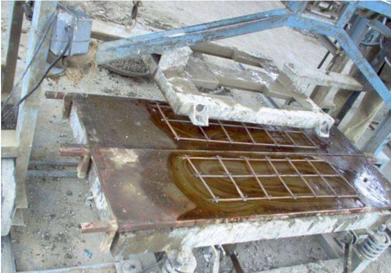
Setting up the trays with reinforcement mesh on plank machine
