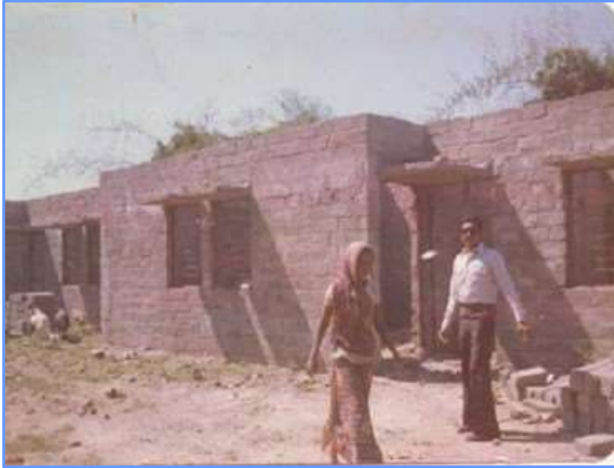
View of stone block masonry housing at Bhopal
