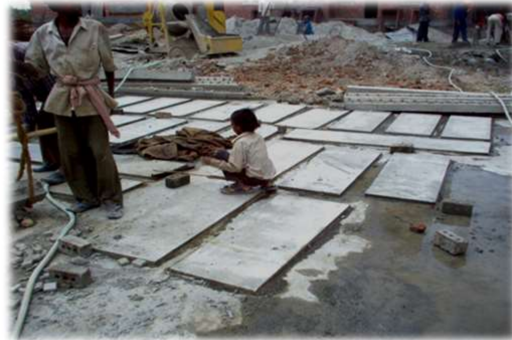
Precast ferro-cement Kitchen platform
