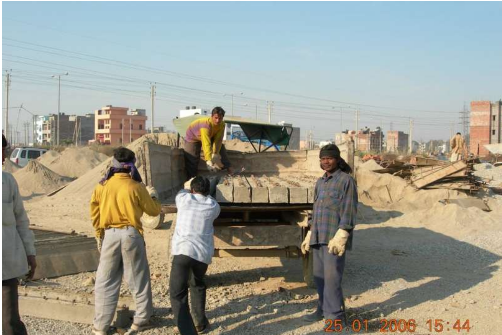
Transporting joists to construction site.
