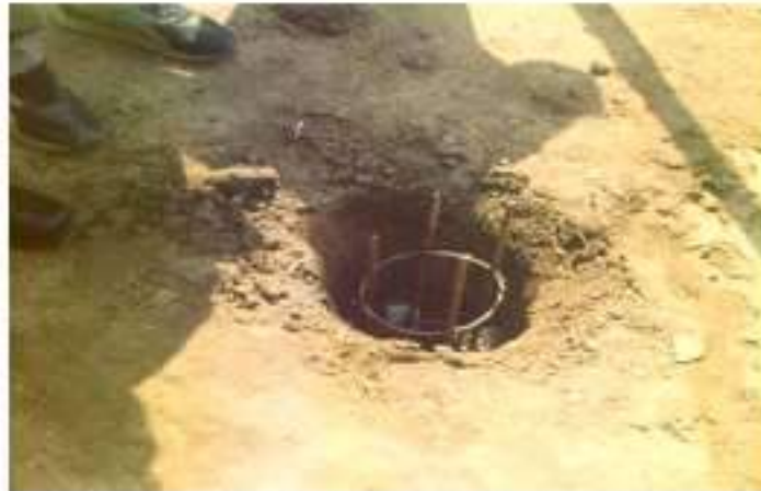
Fig. 2 – Reinforcement Cage in Under-ream Borehole
