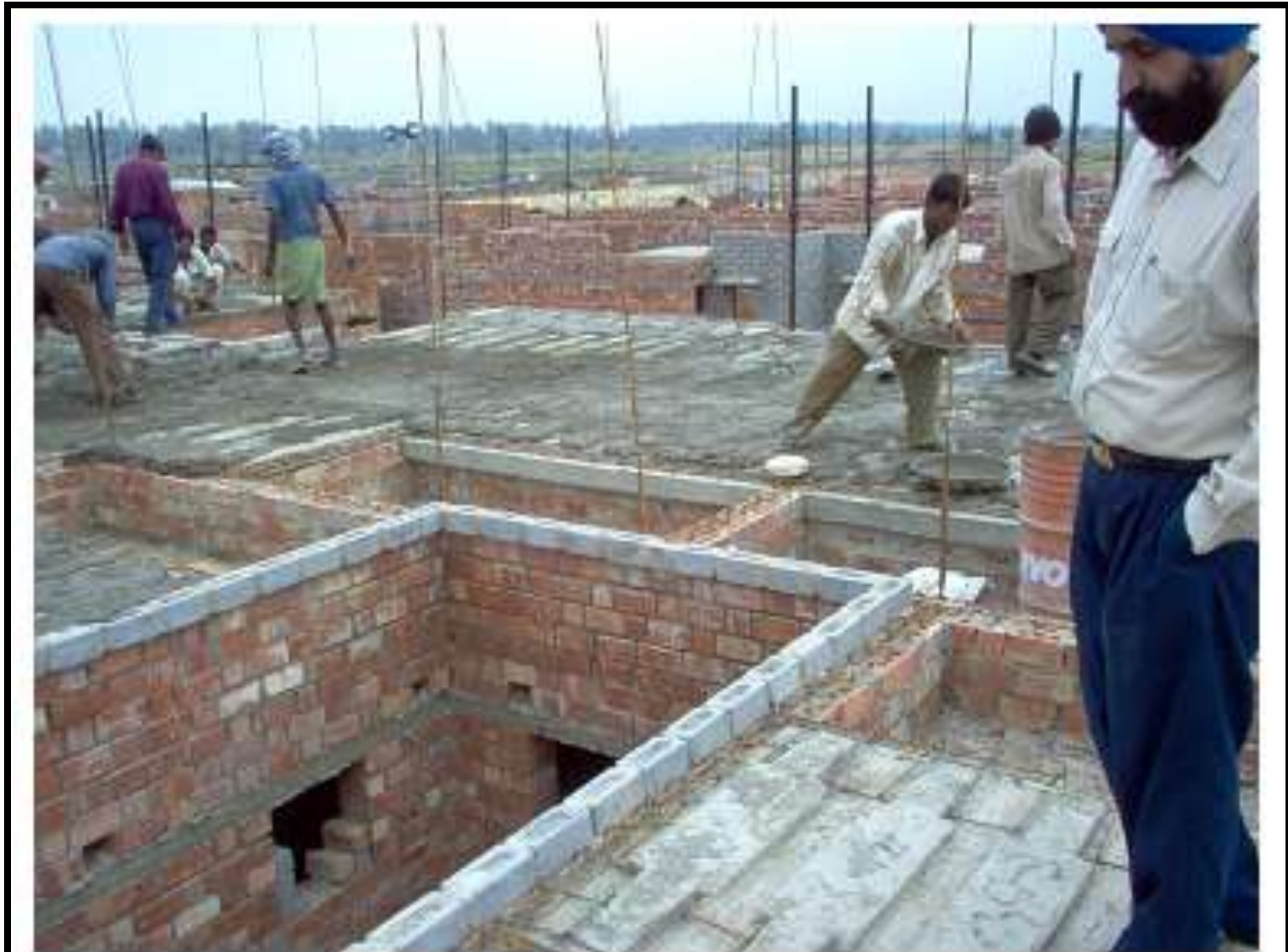
Photograph of roof band
