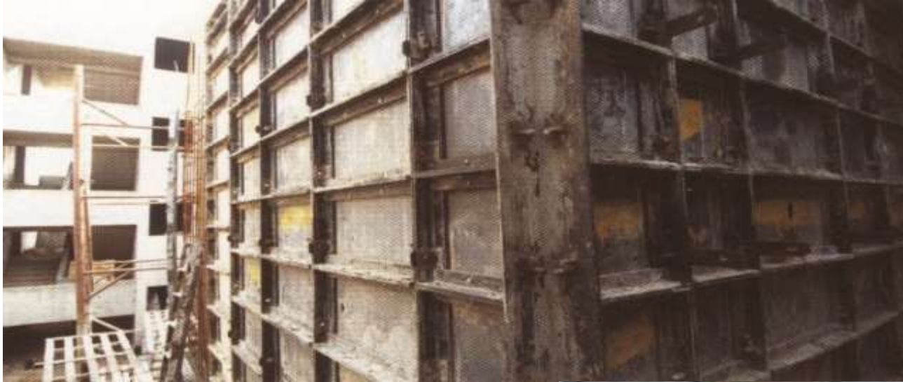
External wall corner Formwork
