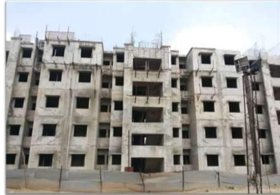
Multistoreyed building in Progress
