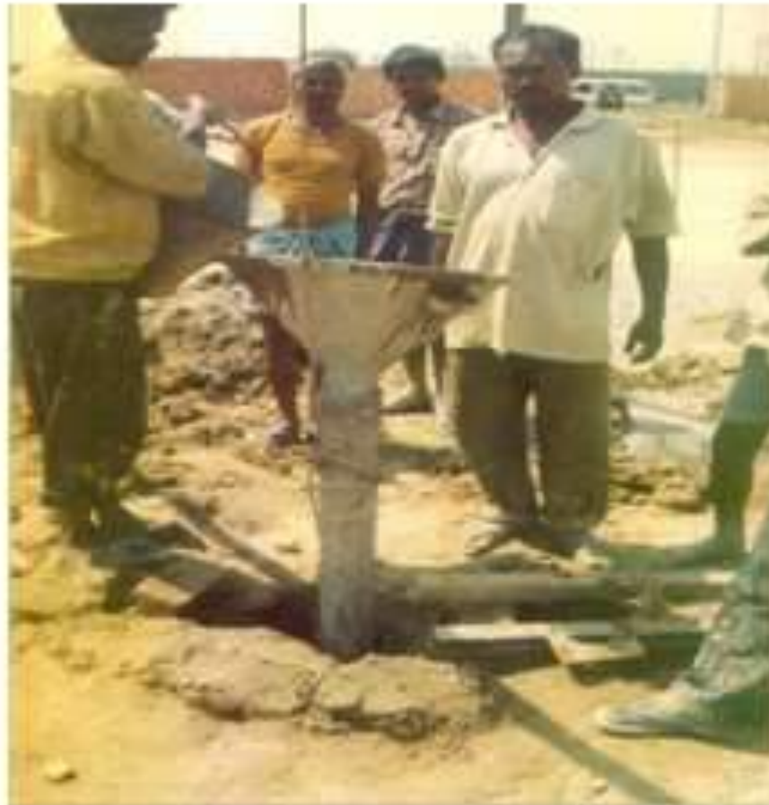
Fig. 1 – Pile Casting through a Tremie
