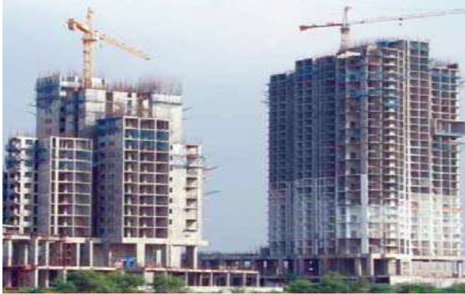
Multistoreyed Building under Construction with Monolithic Technology in Mumbai
