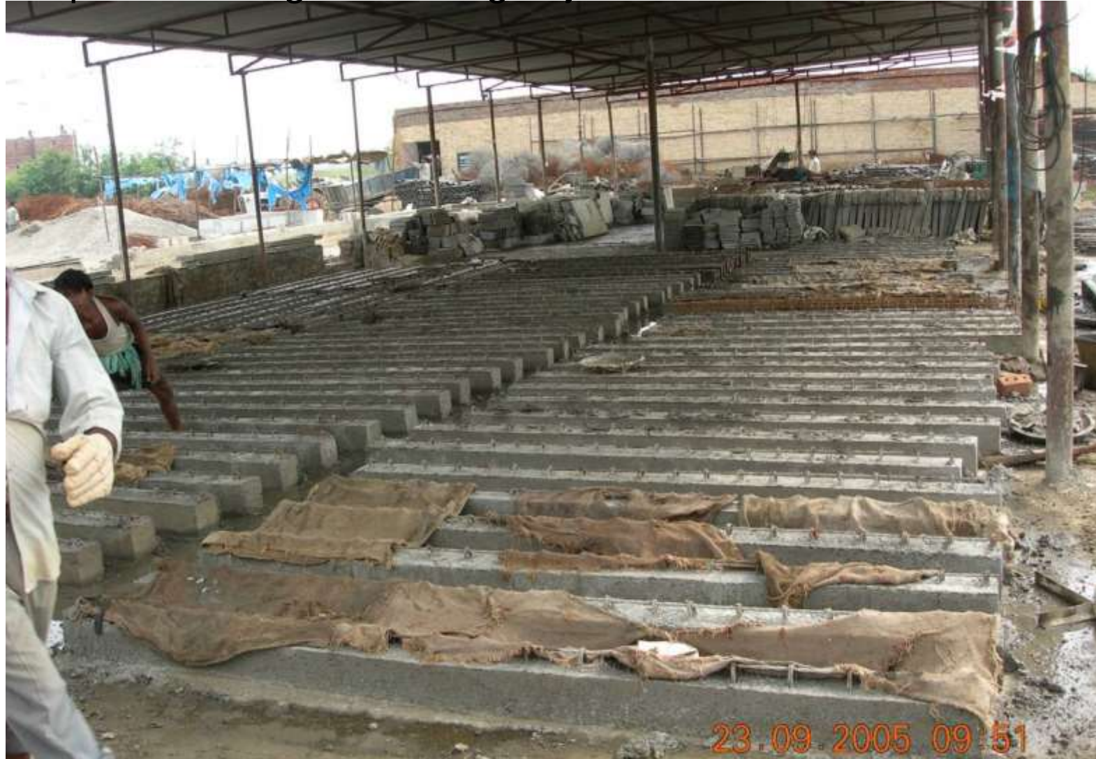
Curing of casted joists.
