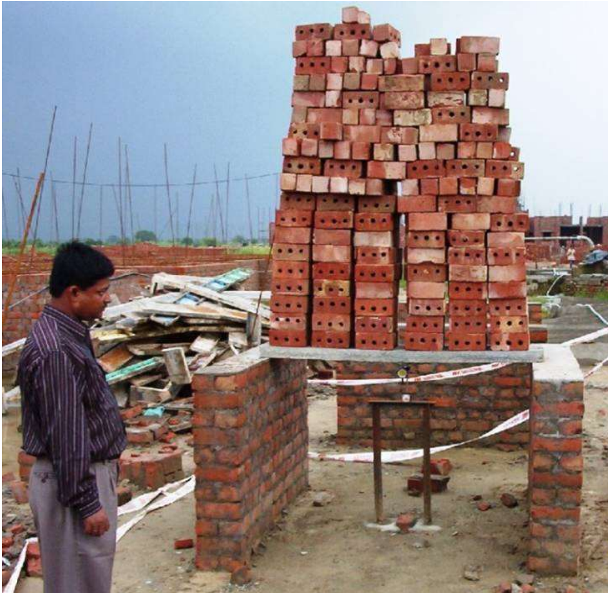
R.C. PLANK LOAD TEST
