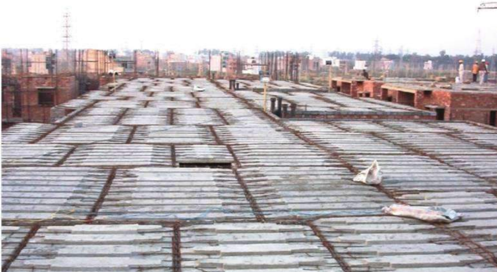
Negative reinforcements in haunches of planks.
