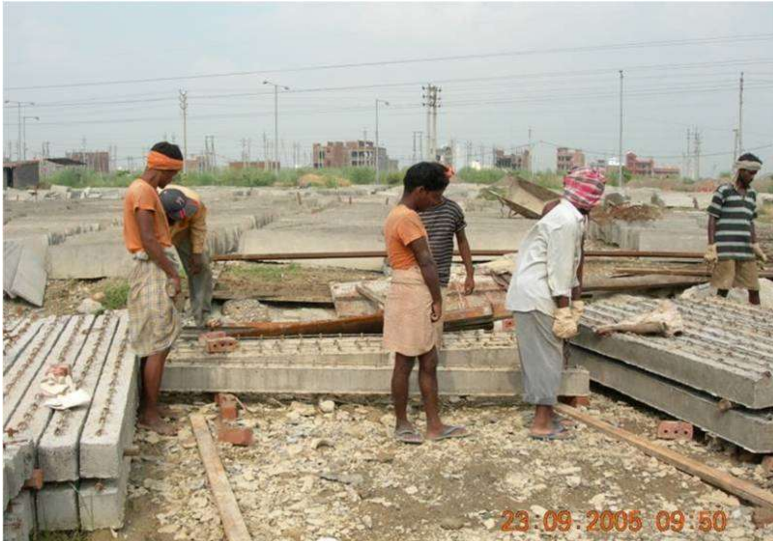
Lifting joists to be taken to construction site.
