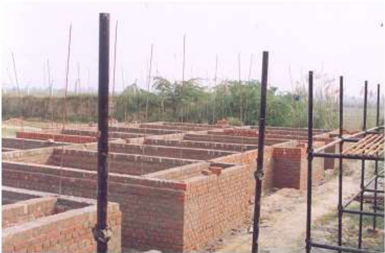
Plinth band & Vertical Reinforcement (for Earthquake Resistance)
