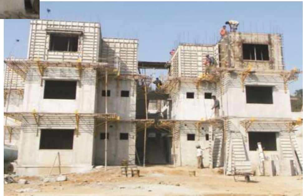
External wall Formwork for Second Floor
