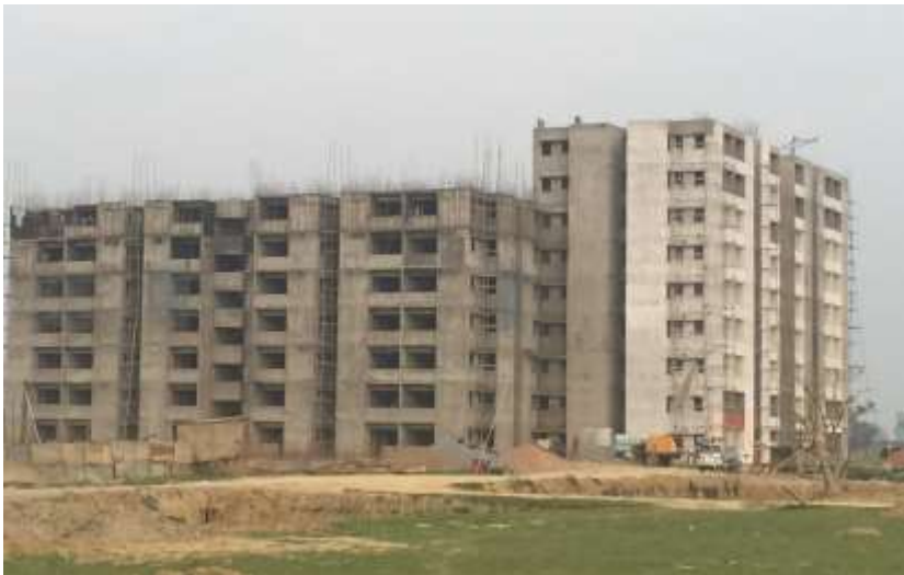
View of multi-storeyed building at Lucknow
