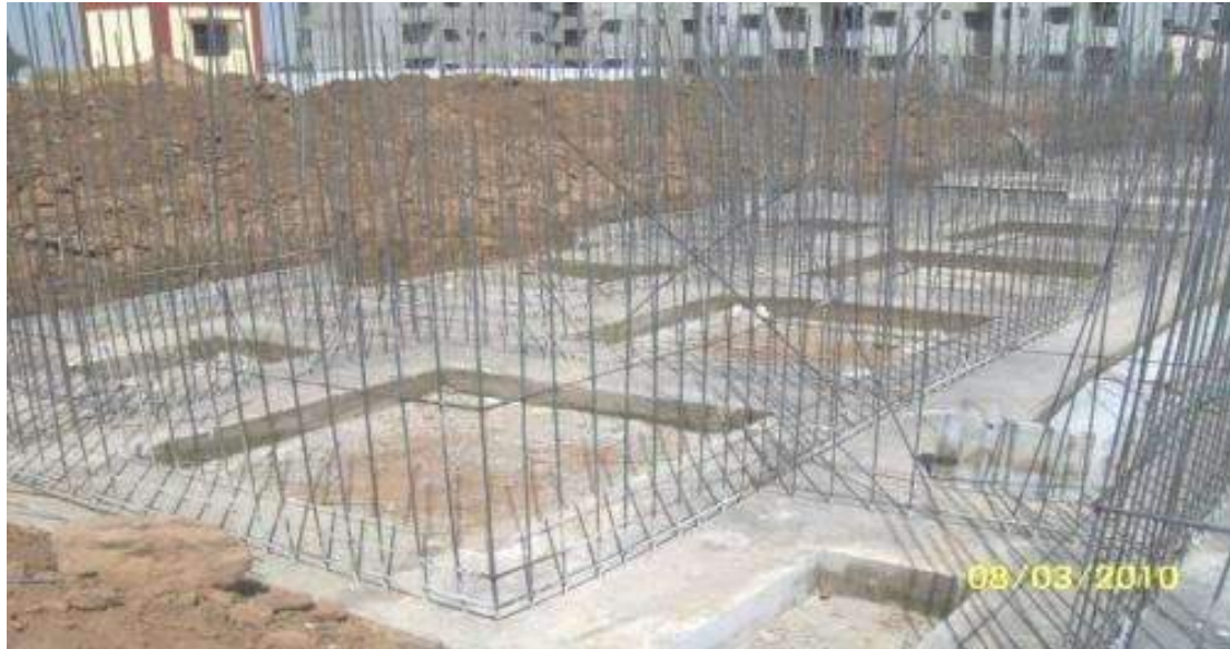
Laying RCC strip foundation with dowel bars and wall reinforcement
