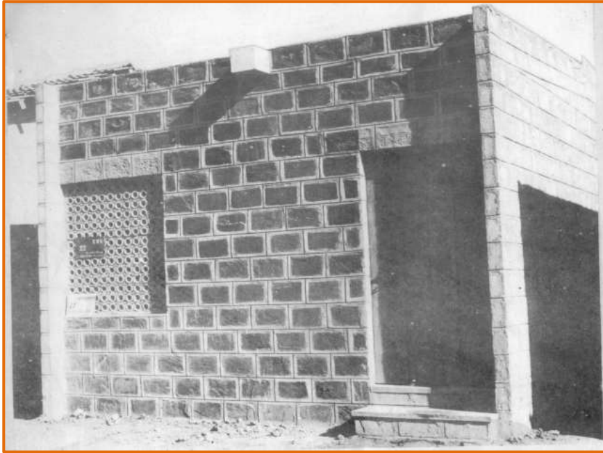
A Building in Housing Rajasthan With Stone Block Masonry
